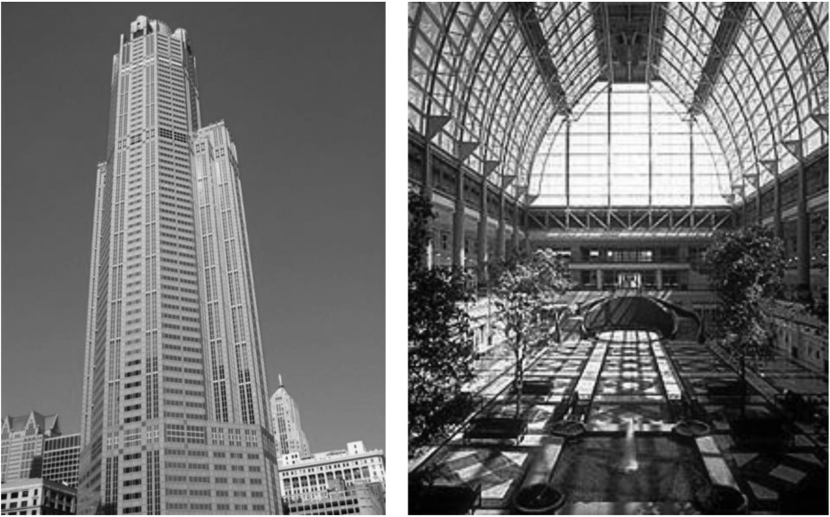
Figure 2. 311 South Wacker Building
