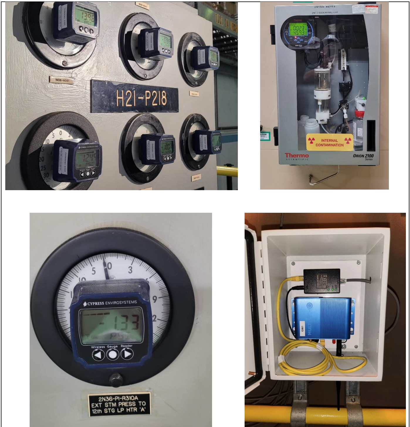
Figure 5 – Installation at Hatch - Operating Nuclear Power Plant
