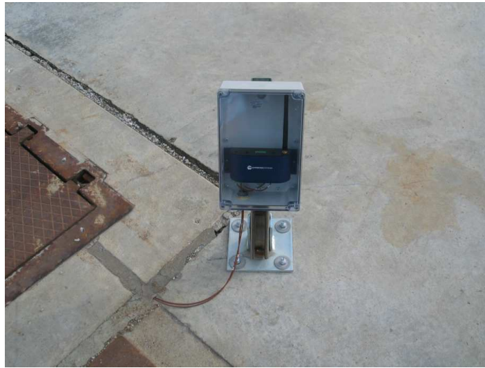
Figure VI – Inaccessible “HOT VAULT” traps at temperatures up to 500F does not hinder getting the condition data of the steam trap back to the Blue Box Server
