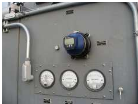
Wireless Magnehelic Reader Monitors Filters and Airflow
