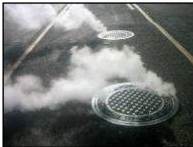
Leaking Traps Waste Energy
