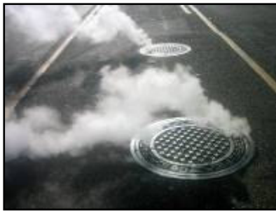
Leaking Traps Waste Energy
