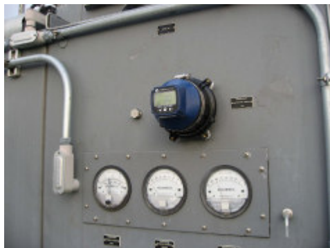
Wireless Magnetic Reader Monitors Filters and Airflow
