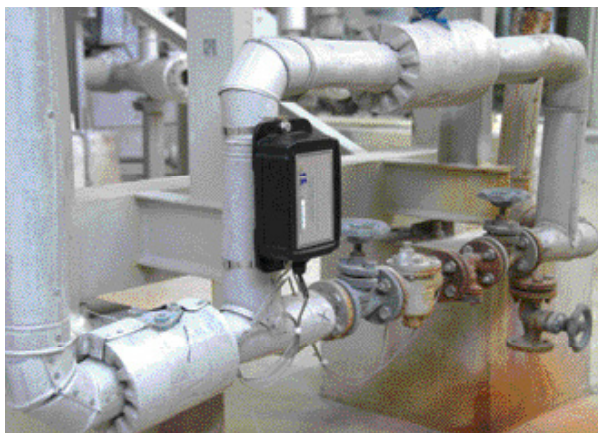
PHOTO B. Wireless steam-trap monitor.
