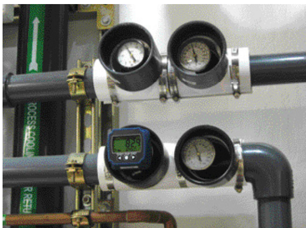
PHOTO A. Wireless gauge reader.
